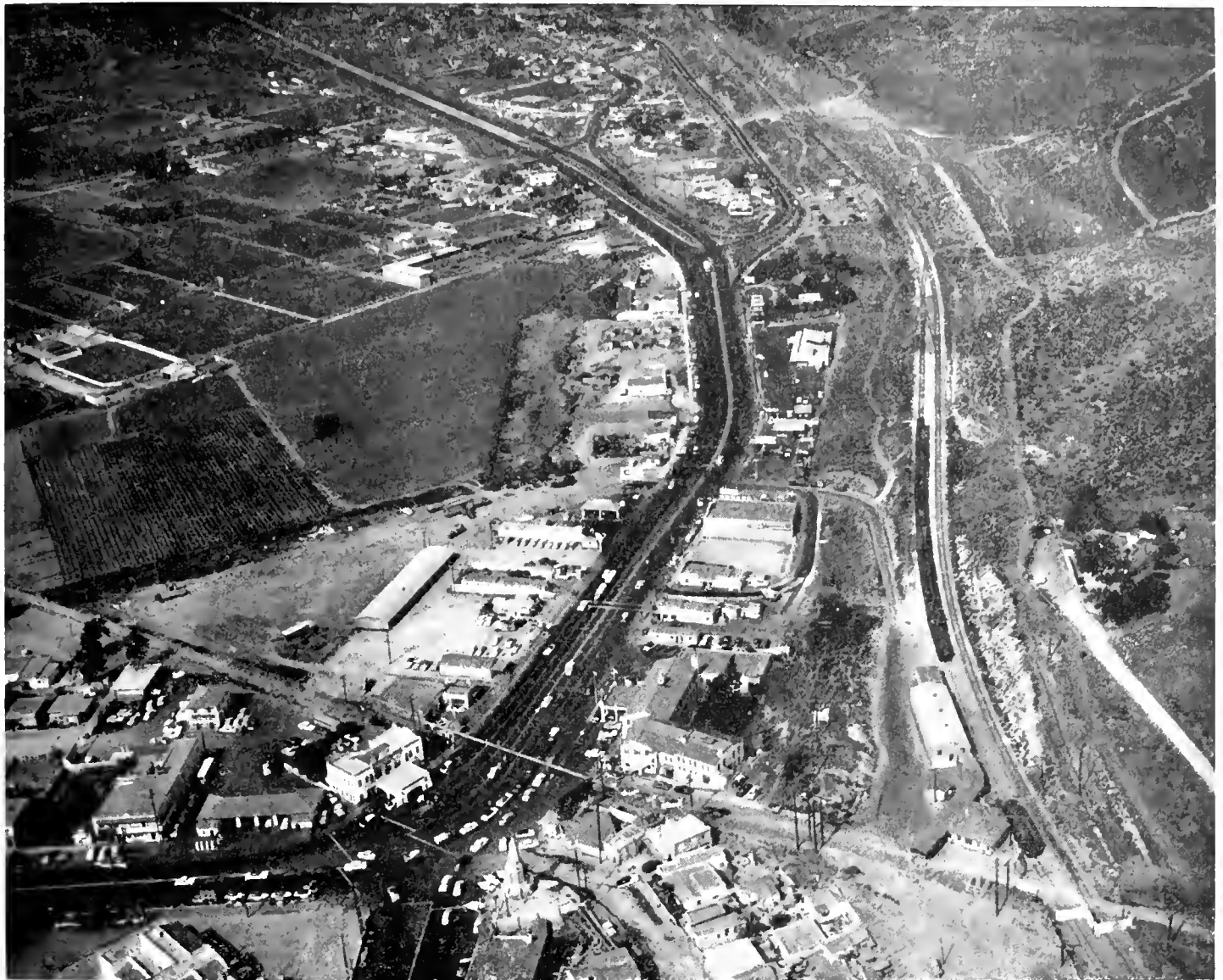
Beginning US 101 and Montgomery Freeway at Mexican border. International Gate in foreground, old US 101 junction in upper right background
